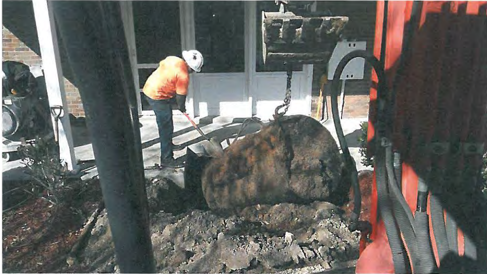
Picture 3:UST 477Dogwood-2 being removed from the excavation.
