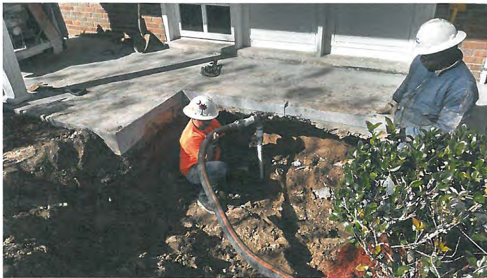
Picture 2: Wastewater being pumped from the tank.
